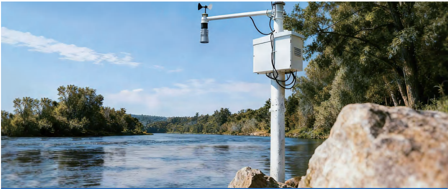
River Water Level Monitoring
