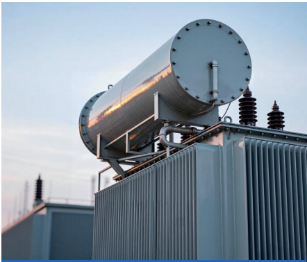
Transformer Oil Conservator Level Monitoring
